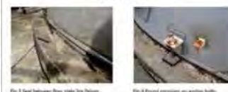
Fig. 3 Seal between floor plate lip failure.
